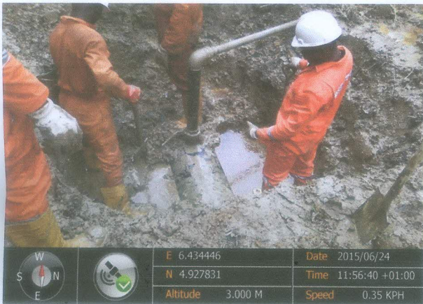
Fig 3 During excavation/ Repair
