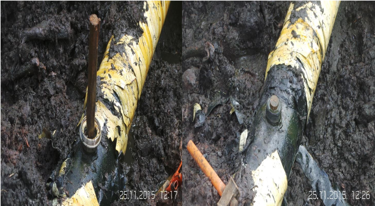
Fig C: Wrapping/Tape coating of incident facility
