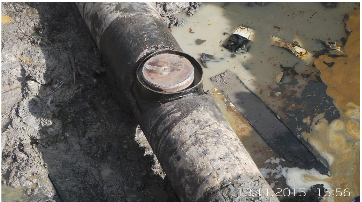
Fig C: Wrapping/Tape coating of incident facility
