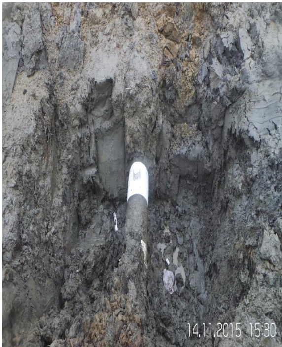
Fig B: Wrapping/Tape coating of incident facility
