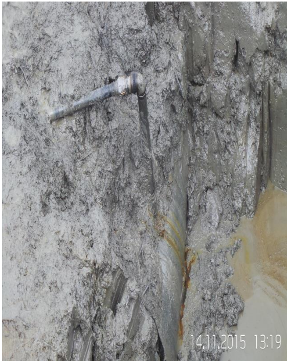
Fig B: Wrapping/Tape coating of incident facility
