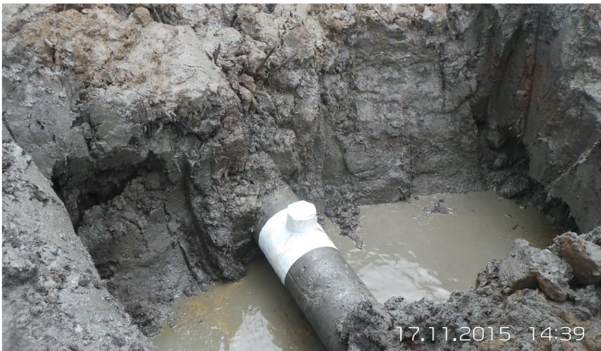
Fig C: Wrapping/Tape coating of incident facility
