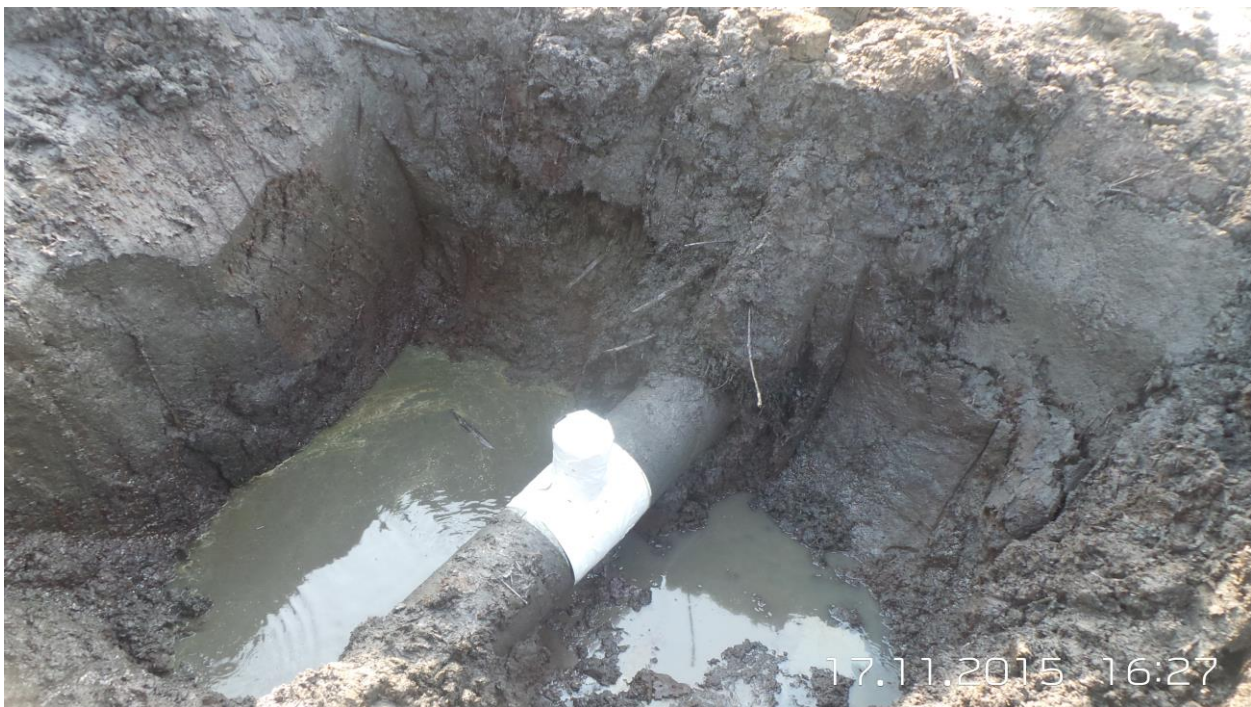
Wrapping/Tape coating of incident facility
