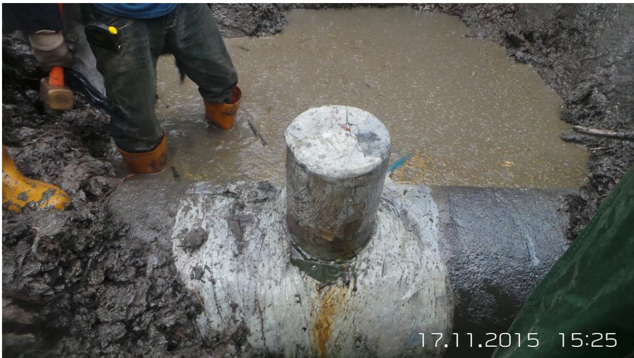
Wrapping/Tape coating of incident facility
