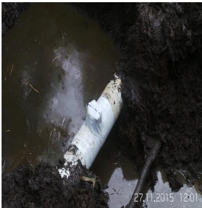
Fig D: Wrapping/Tape coating of incident facility
