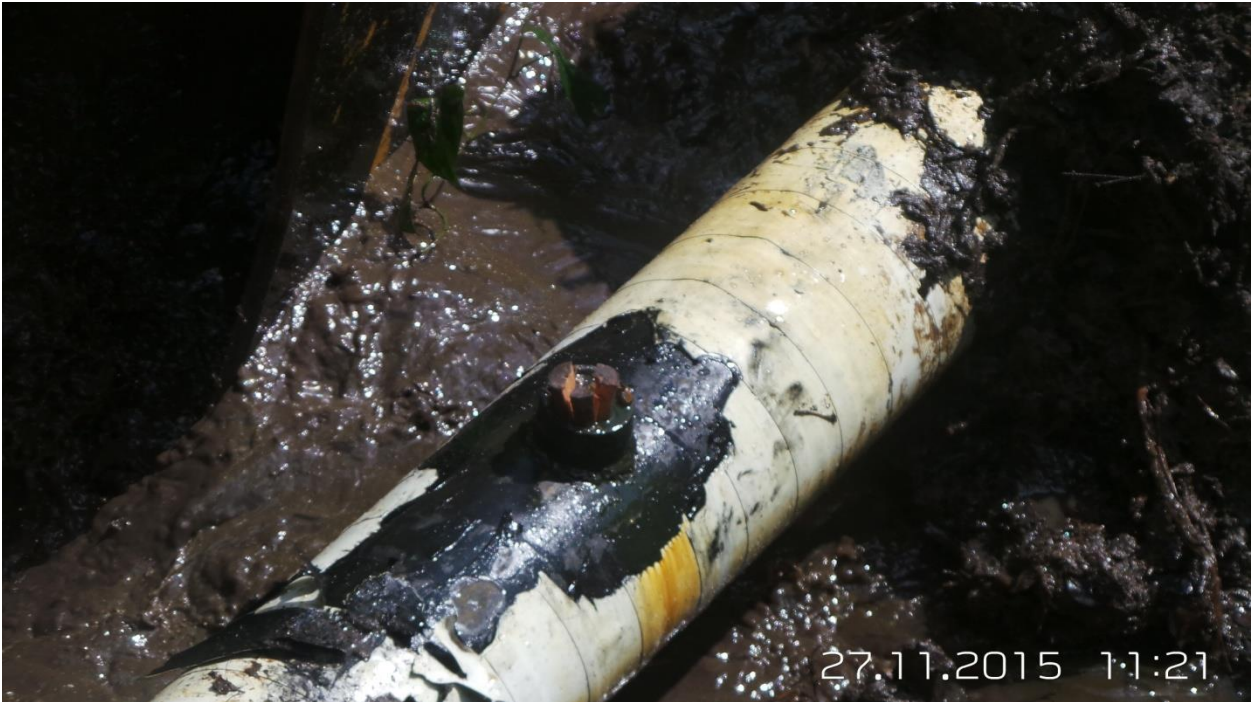
Fig D: Wrapping/Tape coating of incident facility
