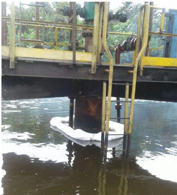
Fig C: Booms directly below the tampered point
