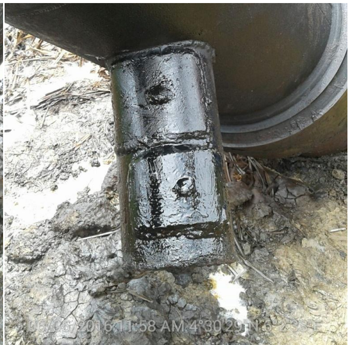
Fig D: The Leak Point after repair
