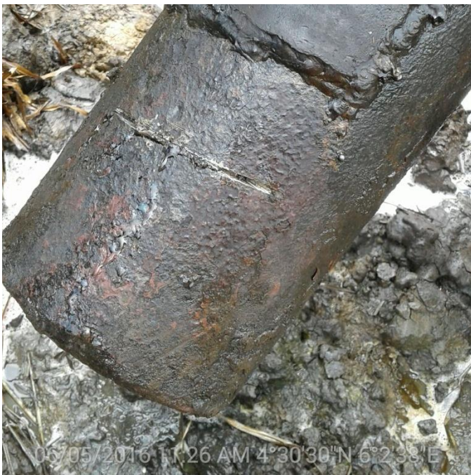
Fig C: Leak point pegged during repair
