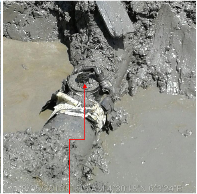
Fig B: The Incident Facility just after excavation.
