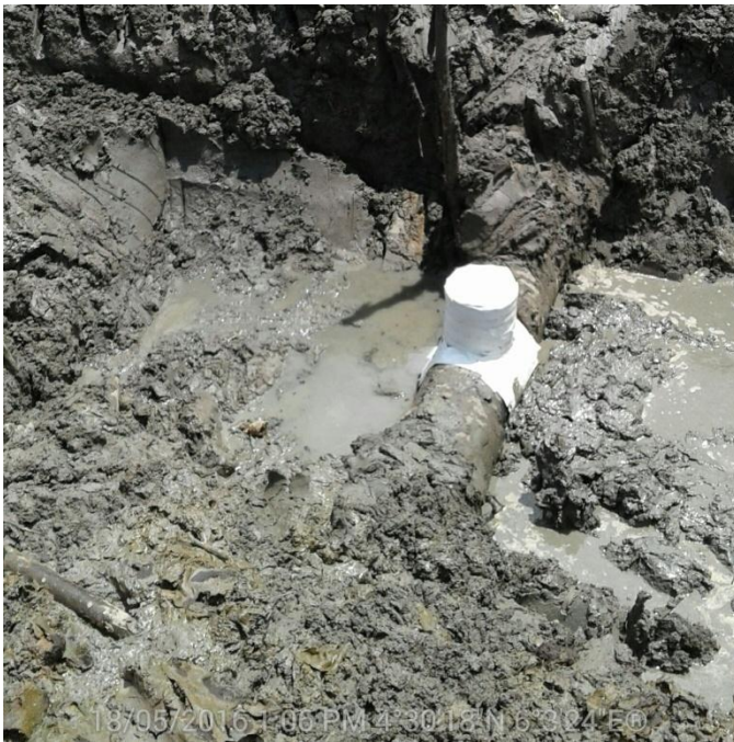
Fig C: The Incident Facility after repair
