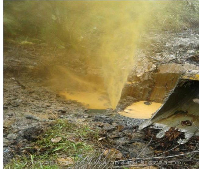
Figure 2: AFTER EXCAVATION 2" Valve found
