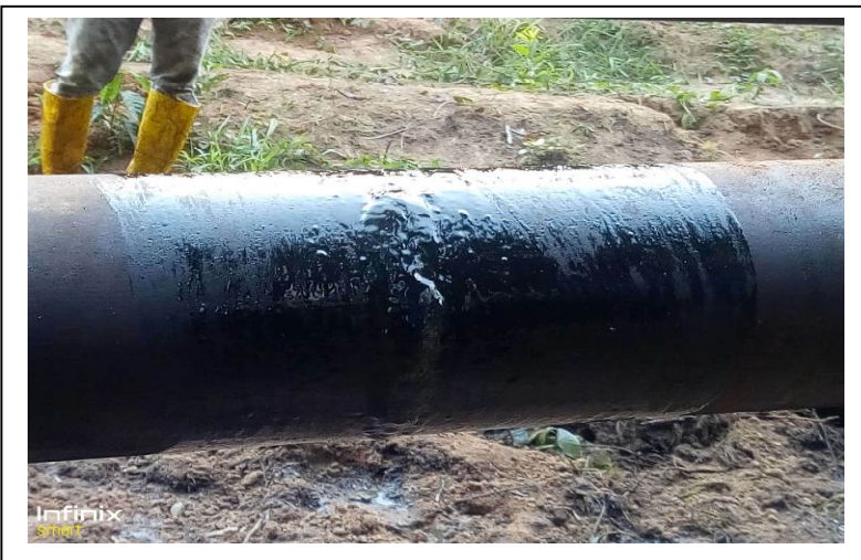
Fig 3: incident point after repairs
