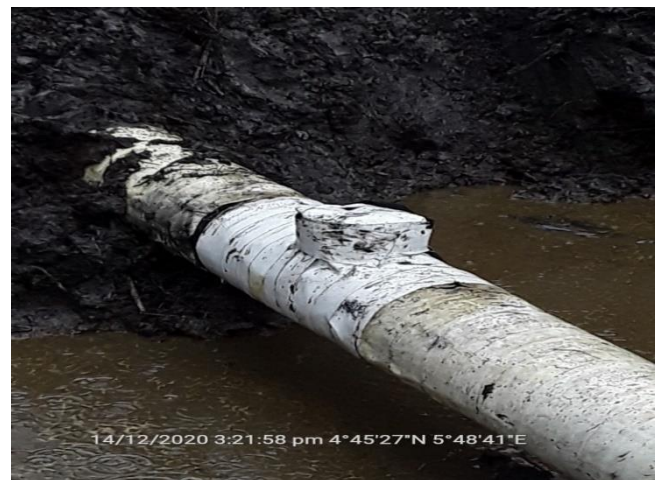
Fig F: Incident Facility immediately after repair
