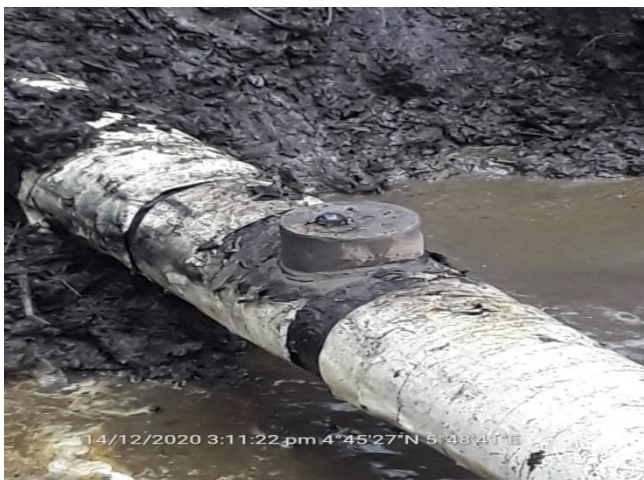
Fig E: Incident Facility during repair
