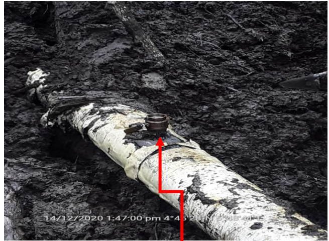
Fig B: Incident Facility shortly after excavation
