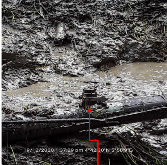
Fig B: Incident Facility shortly after excavation
