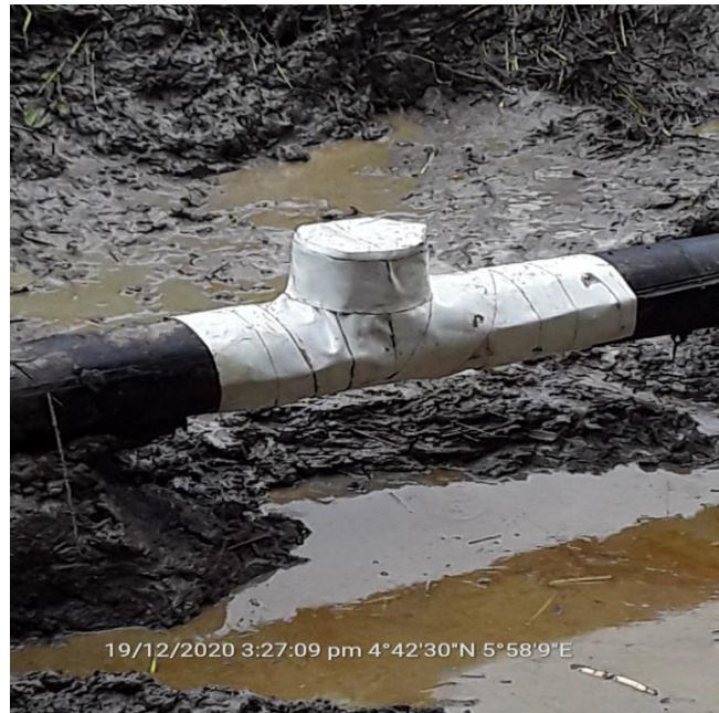
Fig D: Incident Facility shortly after repair
