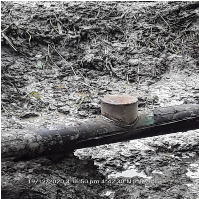
Fig C: Incident Facility during repair
